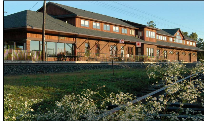
The Bangor depot, after its renovation
