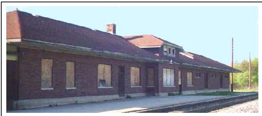
The Bangor depot, before its renovation
